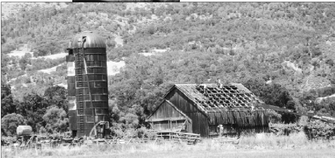
Barbara and Skip are also in the process of moving and restoring a smaller barn and silo that were built on the same property in Potter Valley as the main barn.
